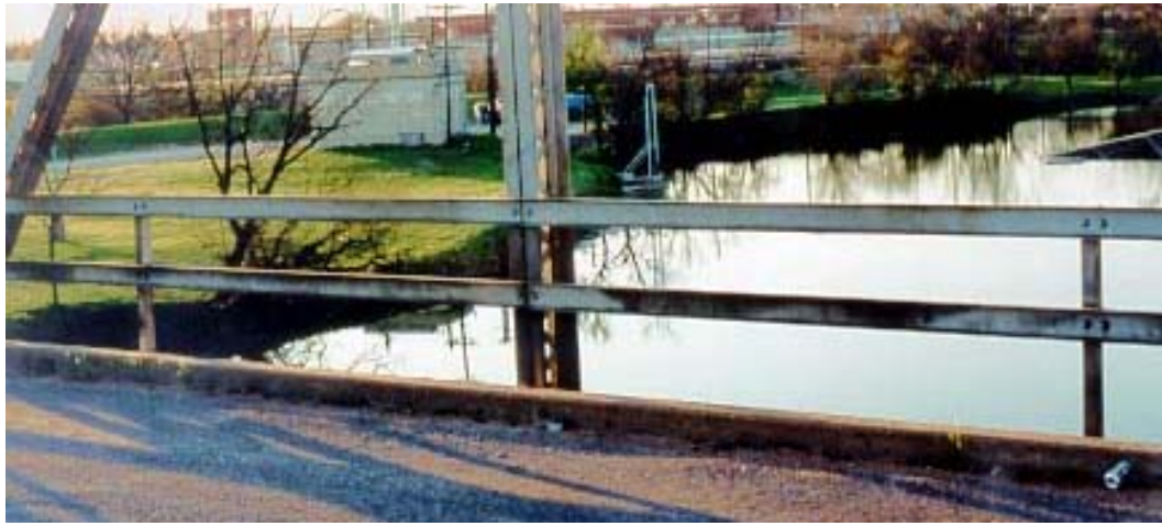
Figure 2.10 Railing attached to vertical and diagonal truss members
