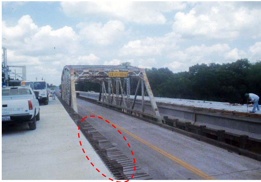
Figure 5.3 Detail showing connecting rebar
