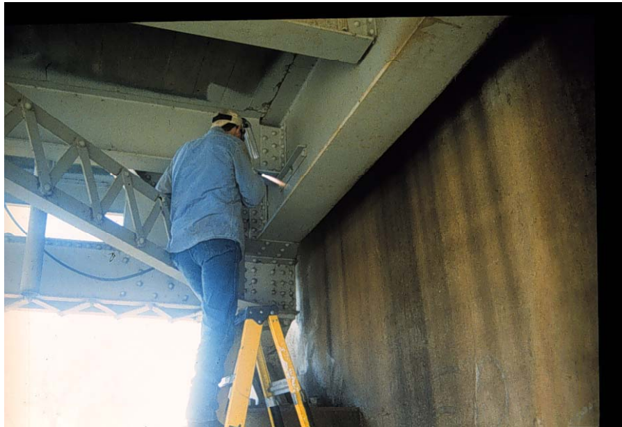
Figure 2.15 Removing the steel sample
