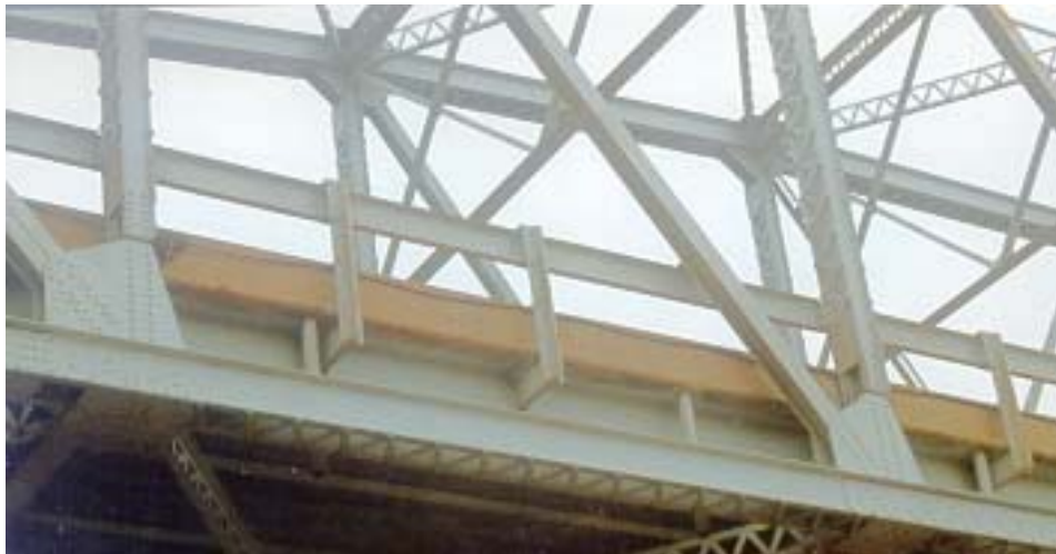
Figure 2.11 Angle attachments of railing to longitudinal stringers
