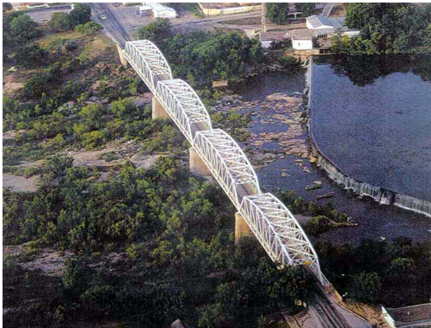
Figure 2.1 Aerial photo of Roy Inks Bridge (photo courtesy of Texas Department of Transportation)
