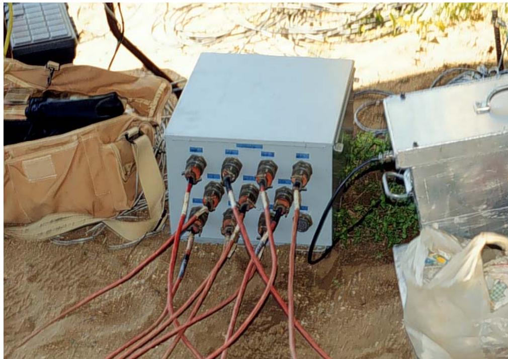
Figure 4.5 CR 9000 data logger
