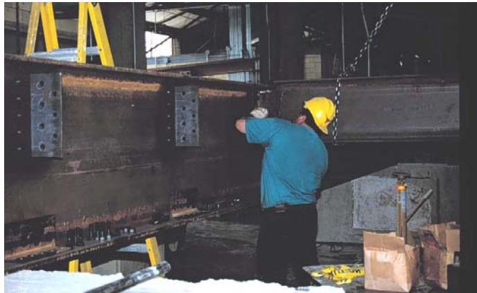
Figure 6.5 Connecting of longitudinal stringer to transverse beam
