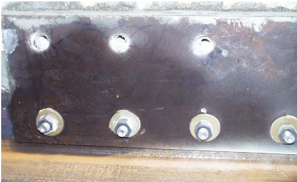
Figure 6.66 Holes drilled up through the plate into the slab
