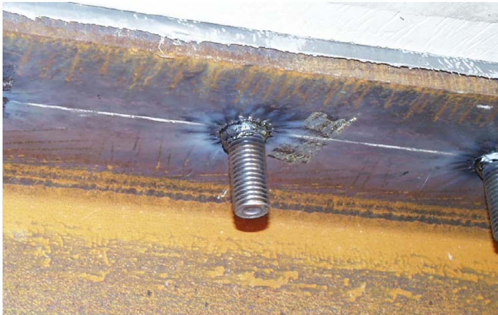
Figure 6.64 Close up view of the threaded stud
