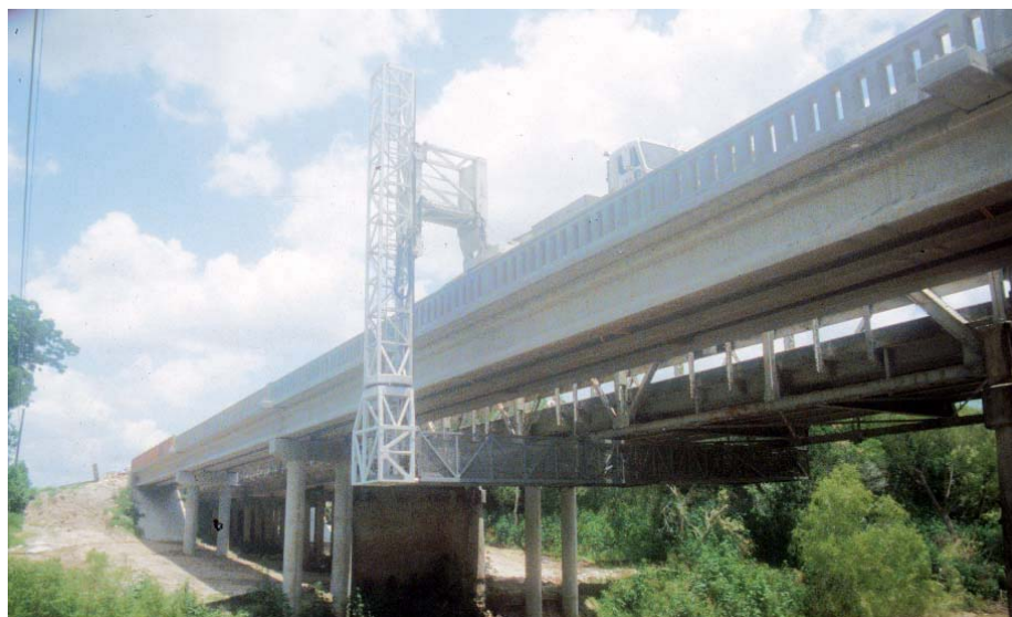
Figure 5.13 Access to bridge deck
