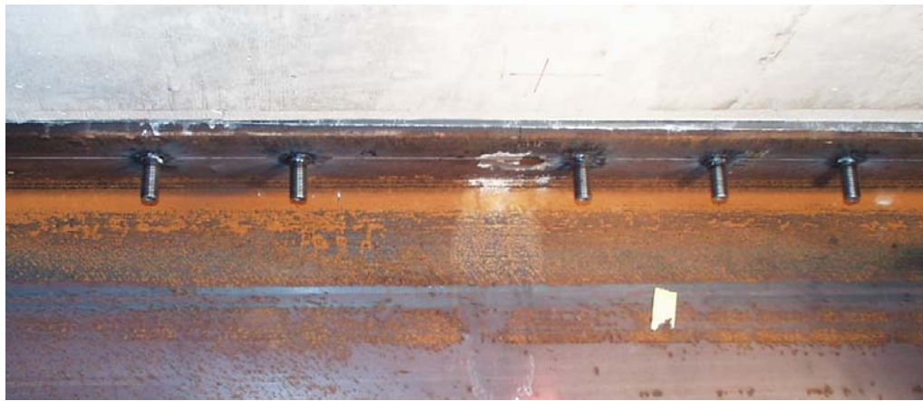
Figure 6.63 Threaded studs welded to the inside top flange of the transverse beam
